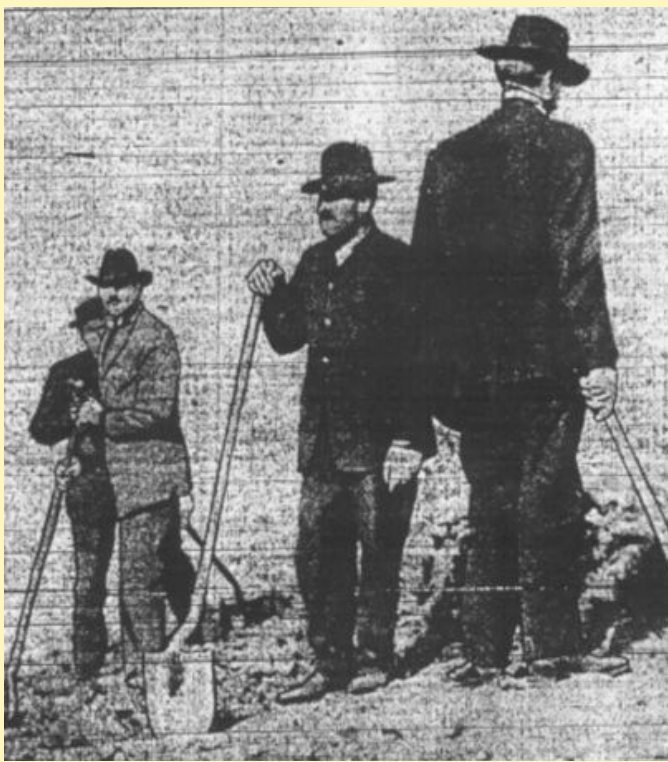
Hard at Work on New County Rockpile Getting Out Rock for Monroe Street Bridge.
